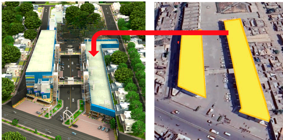
FIGURE 1 Satellite view and physical layout of a commercial shopping plaza.
