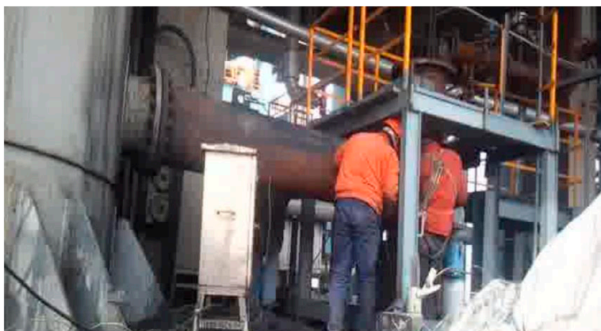
FIGURE 5 Actual monitoring diagram of workers' standing operation in petrochemical plant.
