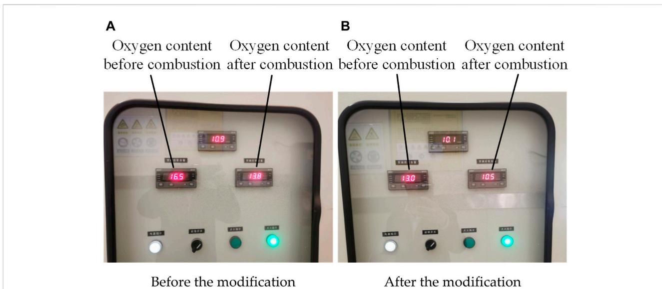
FIGURE 14 (A) Before the modification (B) After the modification. Physical diagram of oxygen content monitoring values at critical points of the combustion furnace system.
