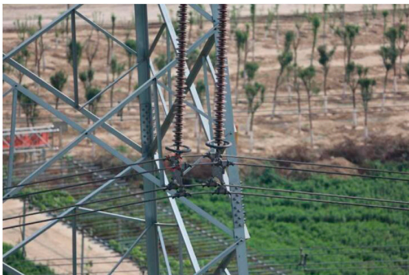
FIGURE 1 Aerial photograph of the original bolts of the transmission line.
