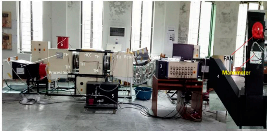
1-Desiccant Wheel 2- Heat Recovery Wheel 3-Data Logger TH- Temperature Humidity Sensor 4-Indirect Evaporative Coller 5-Water Tank 6-Axial Fan 7-Manometer HCC- Heating Coil Chamber
