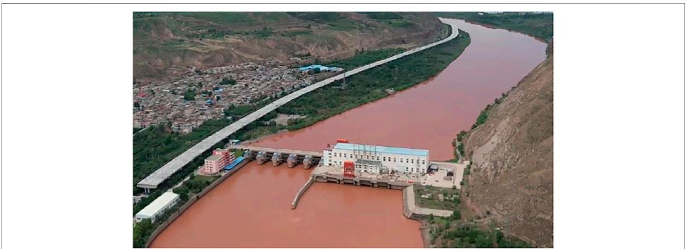
FIGURE 5 | Chajijaxia hydropower station.
