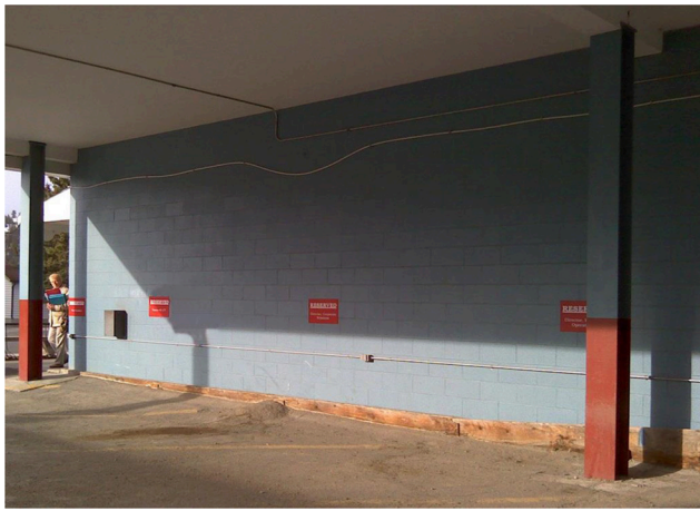
FIGURE 2 | Existing wall selected for retrofit (MacLean and Korn, 2011).
