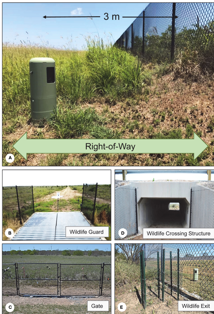
FIGURE 3 Monitoring of mitigation structures along State Highway 100. (A) A total of 10 right-of-way (ROW) cameras were placed on State Highway (SH) 100 in Cameron County, TX facing the chain-link fencing to capture unmonitored wildlife activity occurring along the roadside of the fence. The ROW here is defined as the area between the road and the continuous chain-link fencing that separates the road from the habitat, measuring approximately 5–10 m. Right-of-way cameras were placed approximately 3 m from the chain-link fence. All cameras were checked monthly at which point surrounding vegetation was cleared around each ROW camera. (B–E) In addition to wildlife exits (E) , current monitoring of mitigation structures along State Highway to exists in the form of 16 wildlife guards (B) , 5 wildlife crossing structures (D) , and 16 gates (C) .
