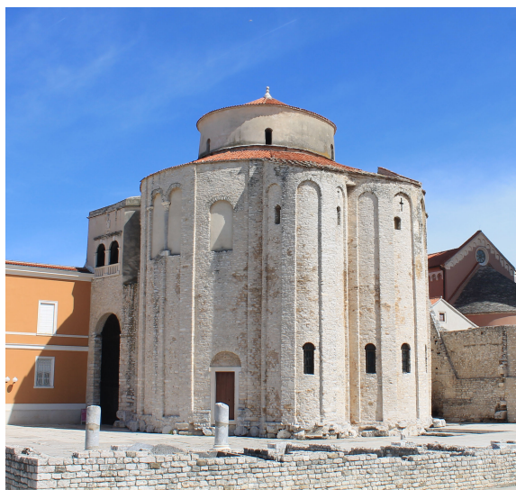
FIGURE 5 Ninth century church of St. Donat in the area of Zadar's Roman forum. Note the heavy use of spolia in its foundation. Restored foundation walls of Roman tabernae in the forum are visible in the foreground. (Photo credit: G. Zaro).
