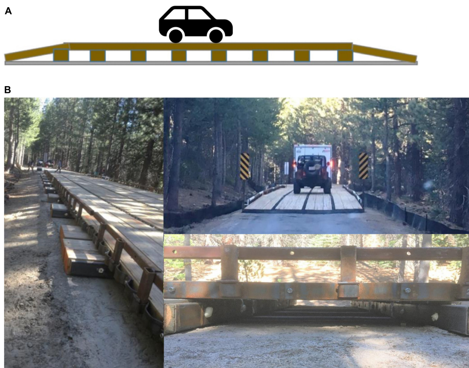
FIGURE 2 Diagram (A) and photos (B) of elevated road segment in Sierra National Forest, Fresno County, CA, USA.
