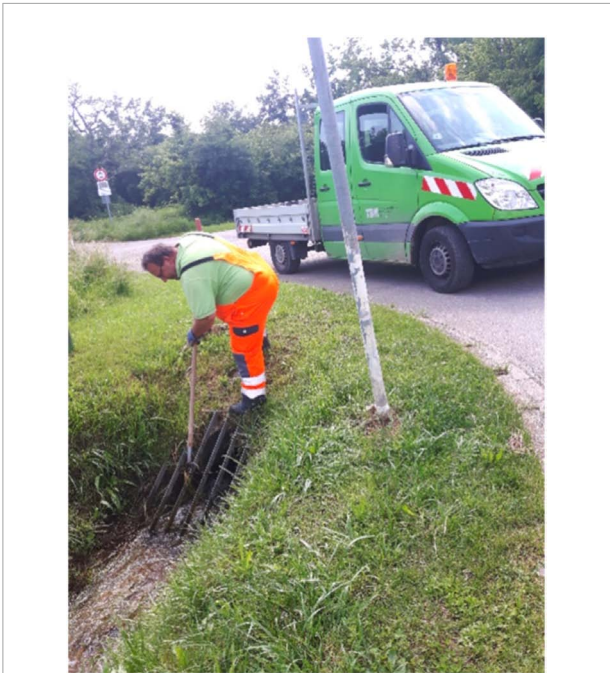
FIGURE 4 Technician cleaning the grid of the entry of the culverted section of an urban stream. Photograph: Karl M. Wantzen.
