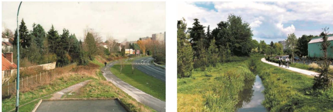
FIGURE 3 The Bièvre before (date) and after (date) daylighting. Photograph: Hervé Cardinal- SIAVB.
