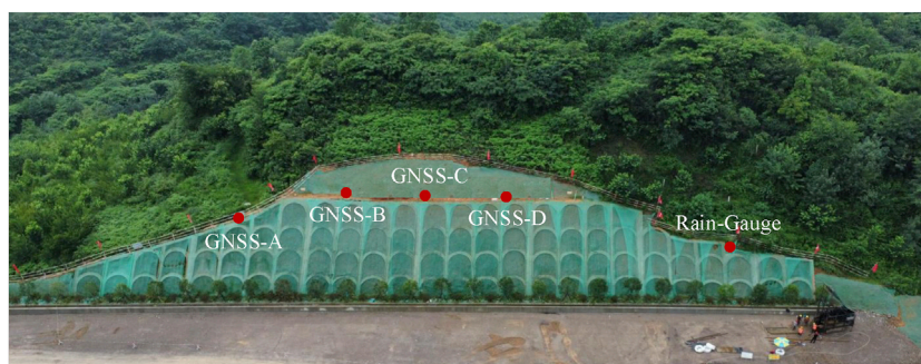
FIGURE 1 Slope site and sensor layout diagram.
