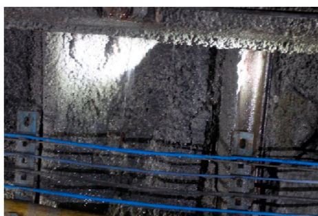
(a) Roof water spraying
