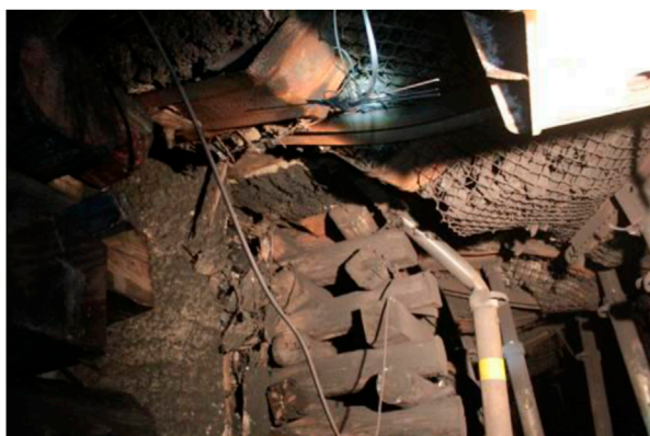
FIGURE 2 Pillar damage.
