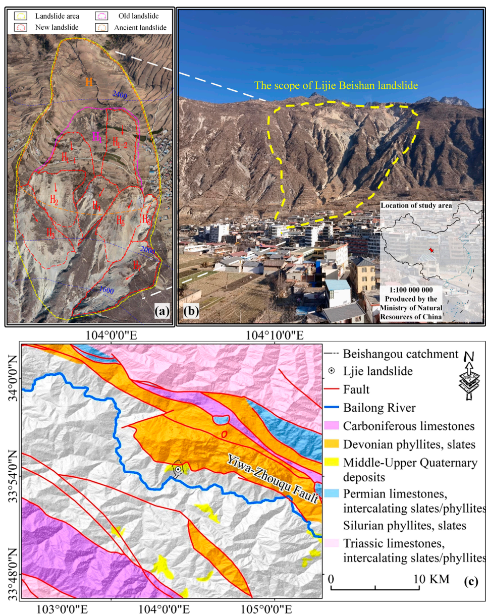
FIGURE 1 Location and field situation of Lijie Beishan landslide.
