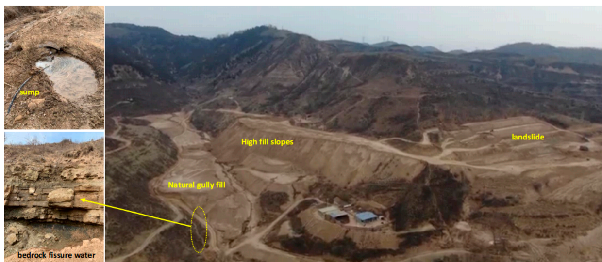
FIGURE 6 Overview of site filling works.
