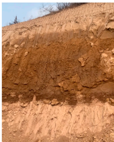
(a) Outcropping of stagnant water at the foot of a steep slope
