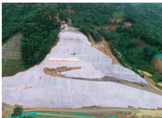
FIGURE 4 Rescue construction for the Naliang slope.
