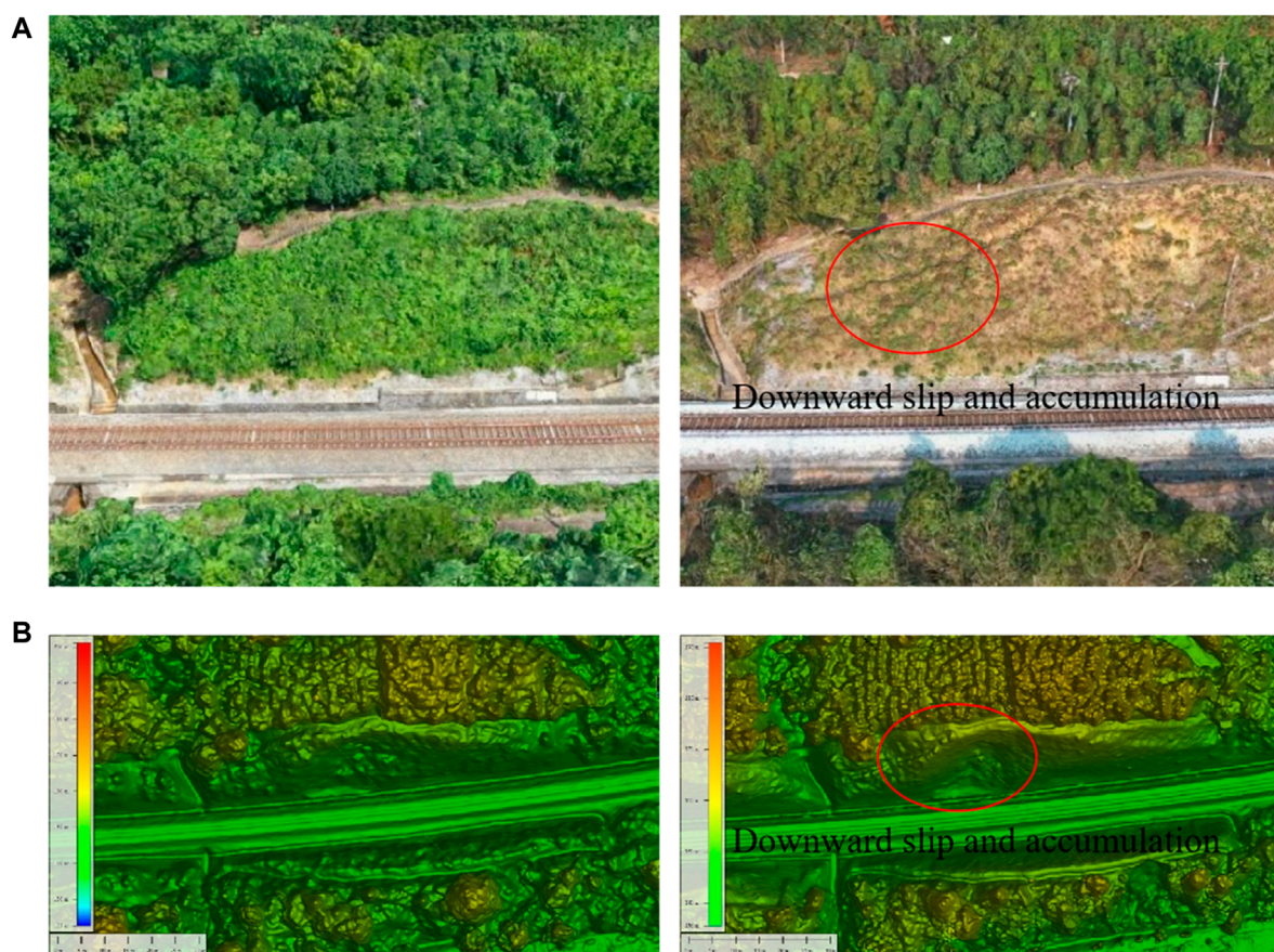
FIGURE 10 Slope protection cycle image of a project section in Hunan and Guangxi. (A) UAV images for June and February of the following year; (B) DSM images for June and February of the following year.
