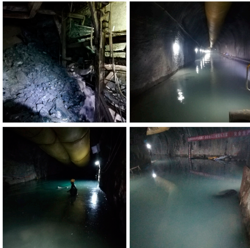
FIGURE 9 The actual situation of the KS2 tunnel water inrush.
