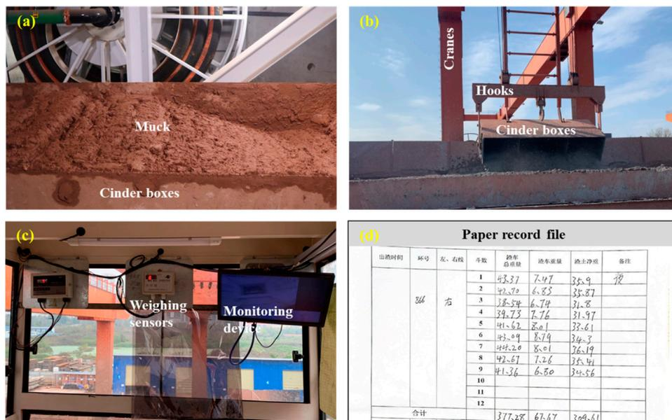
**FIGURE 4** Process of obtaining earthwork excavation amount data: (A) shield tunnel cinder box; (B) gantry crane; (C) control room; (D) paper record file.
