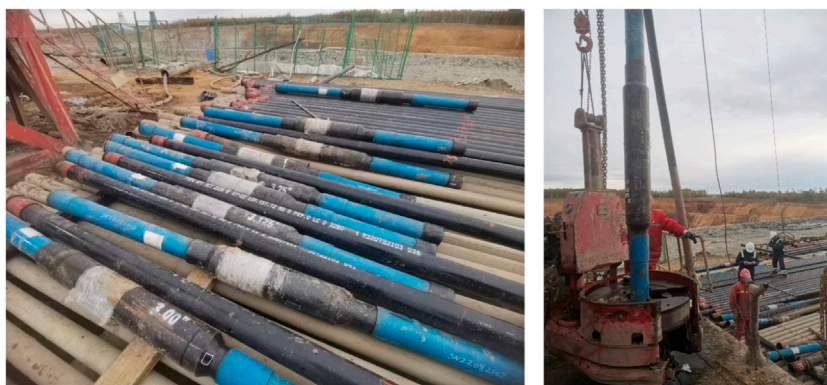
FIGURE 4 The on-site well-logging construction process.
