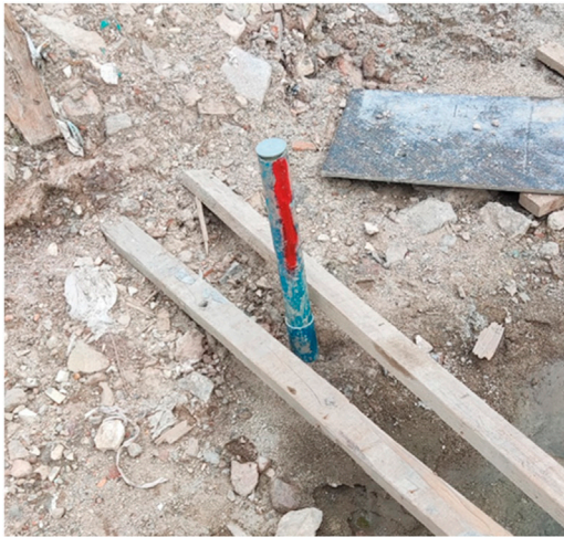
FIGURE 13 Burial of inclined tubes at the construction site.
