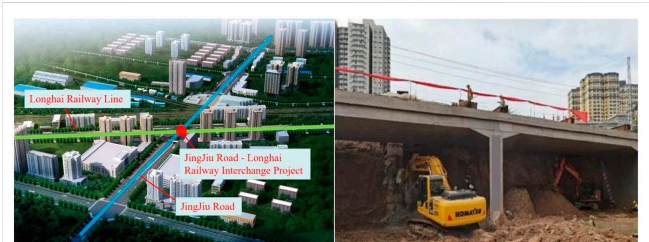
FIGURE 1 Schematic and photograph of the oblique interchange of the Xi'an Jingjiu Lu-Longhai railway project.
