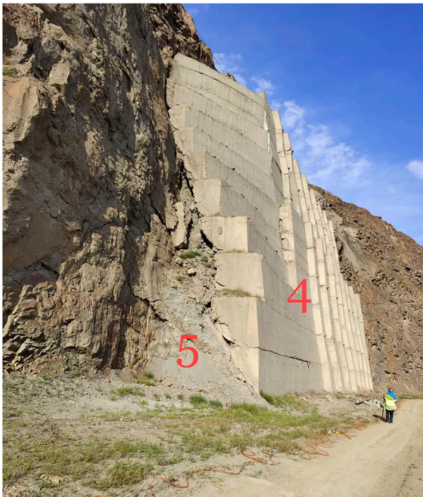
FIGURE 3 Reinforcement area for side slope.
