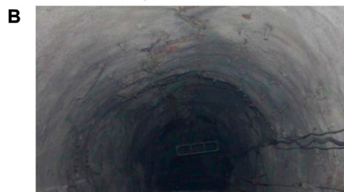
Complete and stable form of roadway after support with CRLD bolt as the main support
