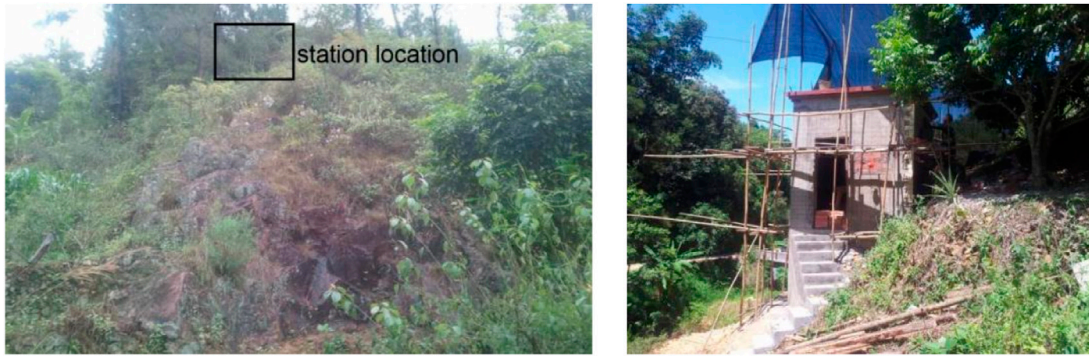
FIGURE 5 Site conditions and working environment of FSLHX station.
