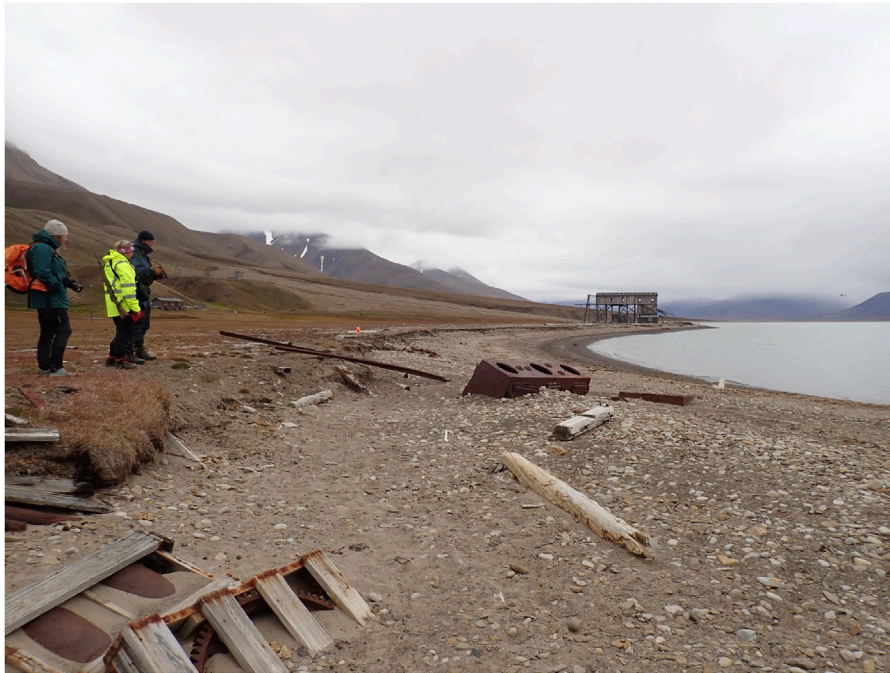
FIGURE 3 The beach at Hiorthhamn, Svalbard, with remains of steam engine and rails on beach. Photo: Vibeke Vandrup Martens, NIKU 2019.
