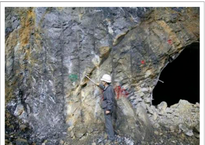
FIGURE 3 | f_{42} fault in the main powerhouse of the right bank.
