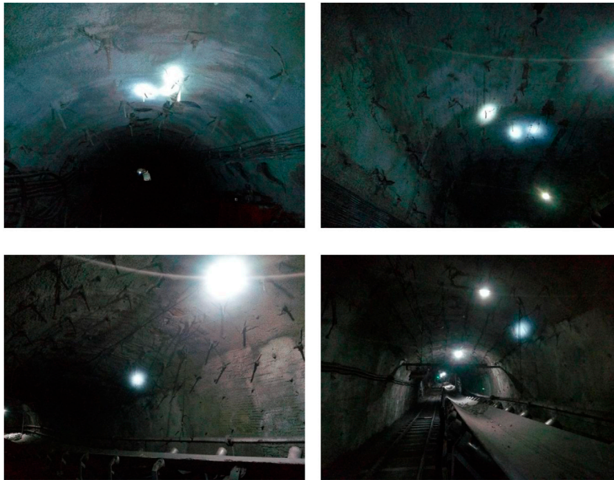
FIGURE 11 | Support effect of the 11 coal belt roadway in the west-east wing of Zhuji.
