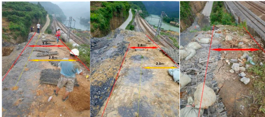
FIGURE 14 | Distance between free face and back of rock wall after each blasting.
