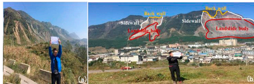
FIGURE 9 Field visit photographs of the landslide in the town of Zongling.
