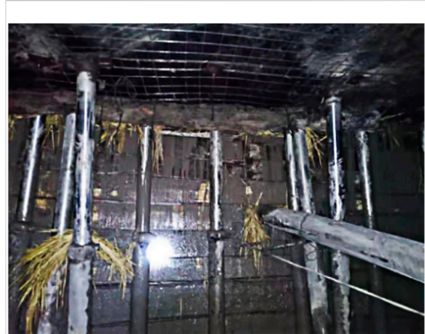
FIGURE 7 Design and construction of a paste baffle.
