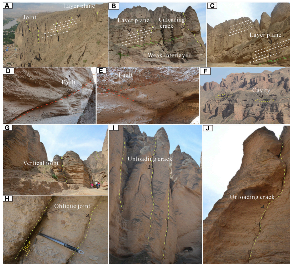
FIGURE 4 | Structural plane types and combination characteristics of typical rock slopes in the study area. (A) Layer plane and joint; (B,C) layer plane, joint, and weak interlayer; (D,E) fault; (F) cavity; (G,H) vertical and oblique joints; and (I,J) unloading fracture.
