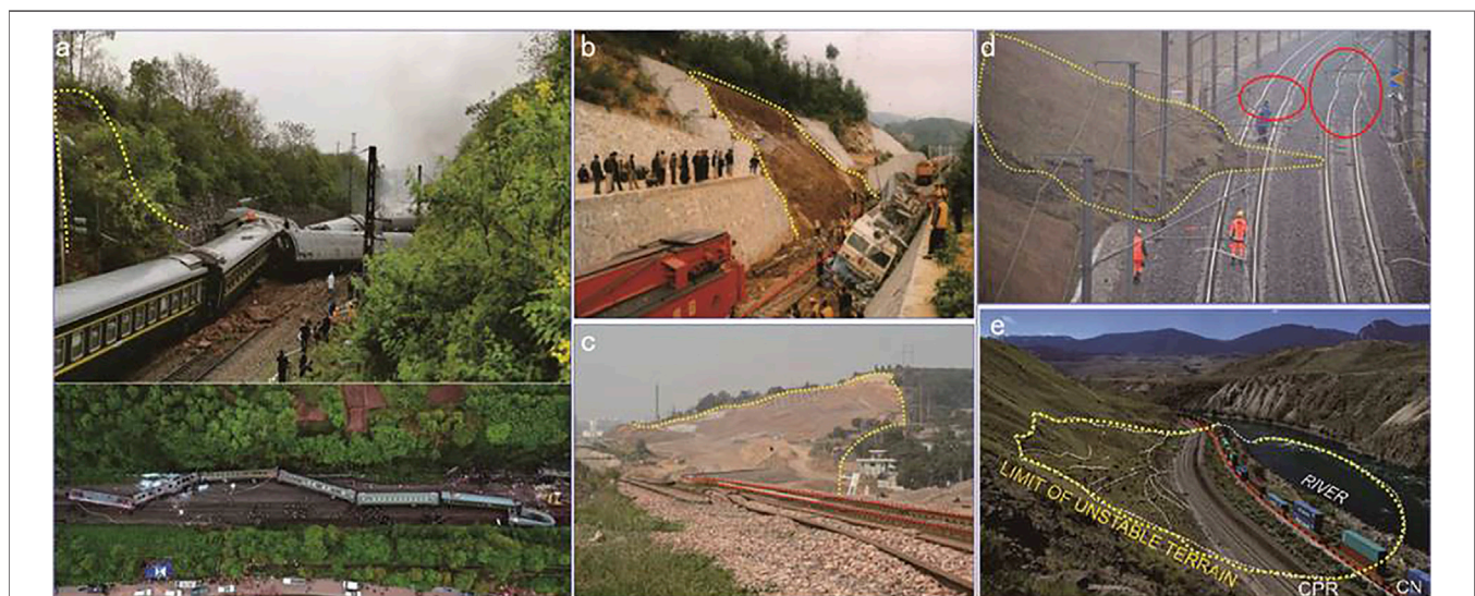
FIGURE 2 | New geological hazards induced by vibration, rainfall, or the coupling effect. (A) Landslide in the Yonghua section of the Beijing–Guangzhou Railway. (B) Typical landslides along a heavy-load railway in Shanxi. (C) Landslide along the Yang-Da Railway (Wang et al., 2021). (D) Landslides along the section close to Strasbourg at the France and Germany border as TGV (Train A Grande Vitesse) is approaching ( https://www.sohu.com/a/377989394_100016456 ). (E) Landslides along the railway near Ashcroft, Canada (Huntley et al., 2019).
