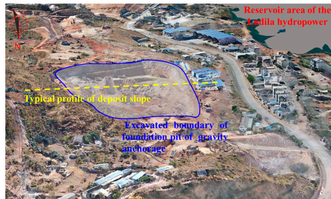
B Excavated boundary of foundation pit of gravity anchorage
