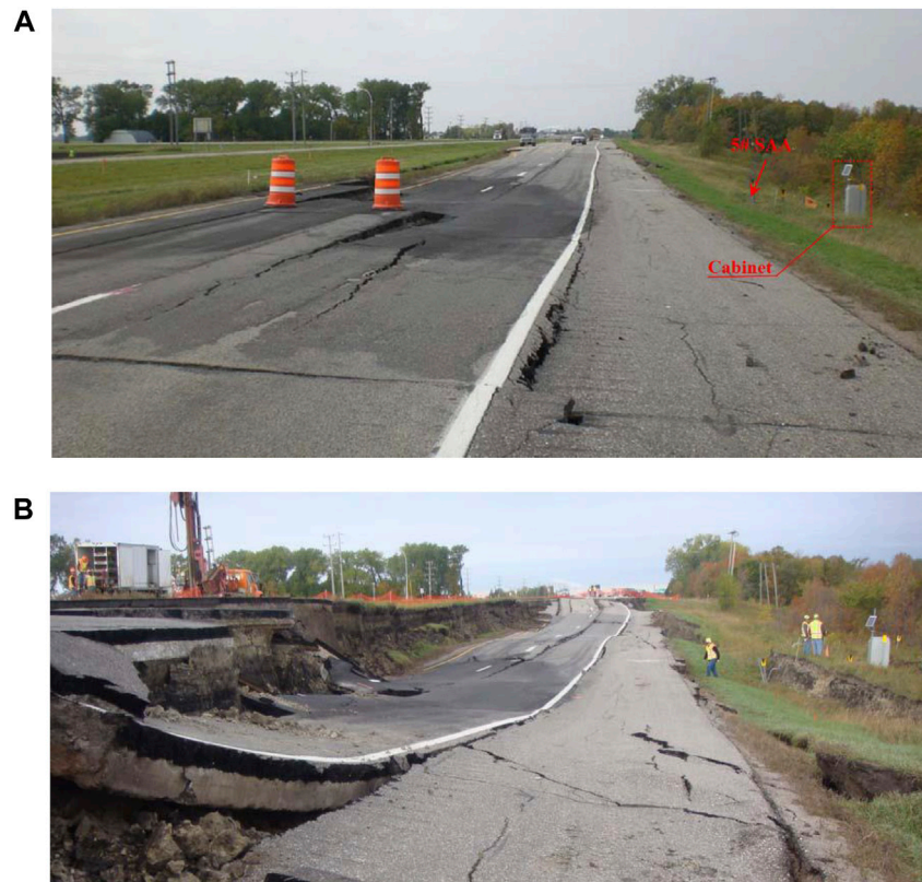
FIGURE 4 | Macroscopic deformation (A) before sliding and (B) after sliding. The 5# SAA and 4# SAA are located about 4.57 m upward and downward from the cabinet, respectively (Modified from Dasenbrock, 2010.)
