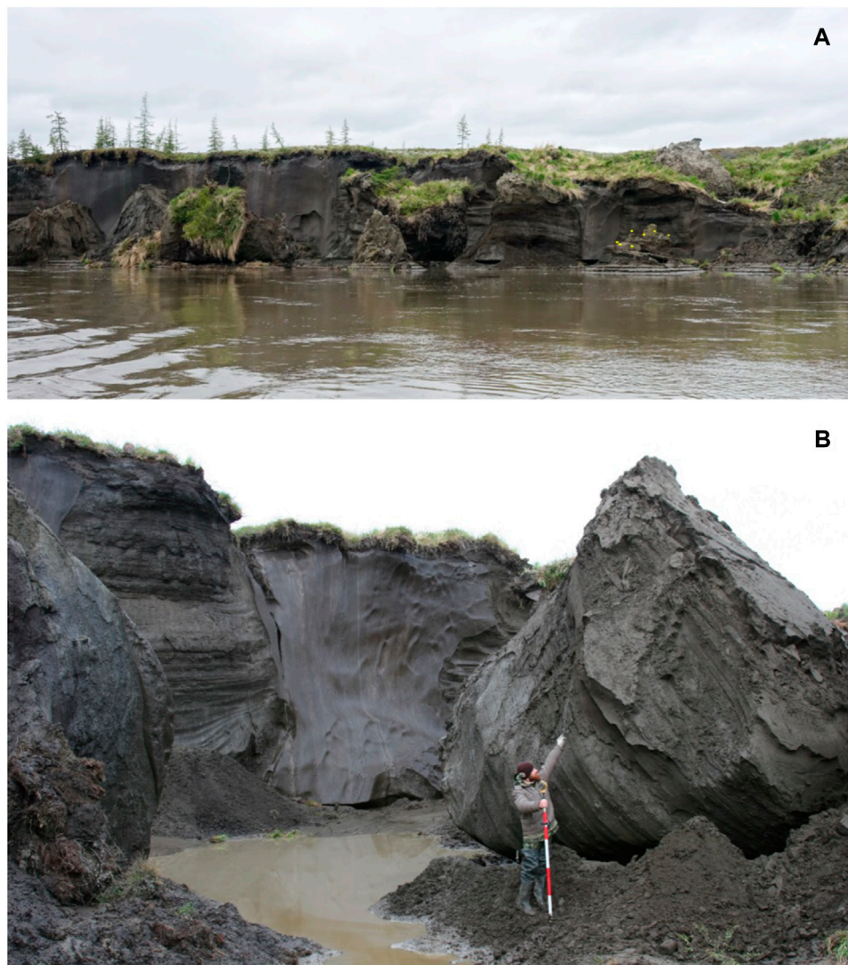
FIGURE 13 | Thermal erosion of the area in the Northern Point area of the Yana site complex: (A) - block collapse at the left bank of the Yana River due to continuously high water stand (collapse zone in between Northern Point and Area B of the Yana site; yellow flags seen in the lower right corner mark the western border of the excavation area); (B) - a cultural layer incorporated in the collapsed blocks, its position is indicated by I.G. Kovaltsov (excavations of 2016). Photo: E.Y. Pavlova.
