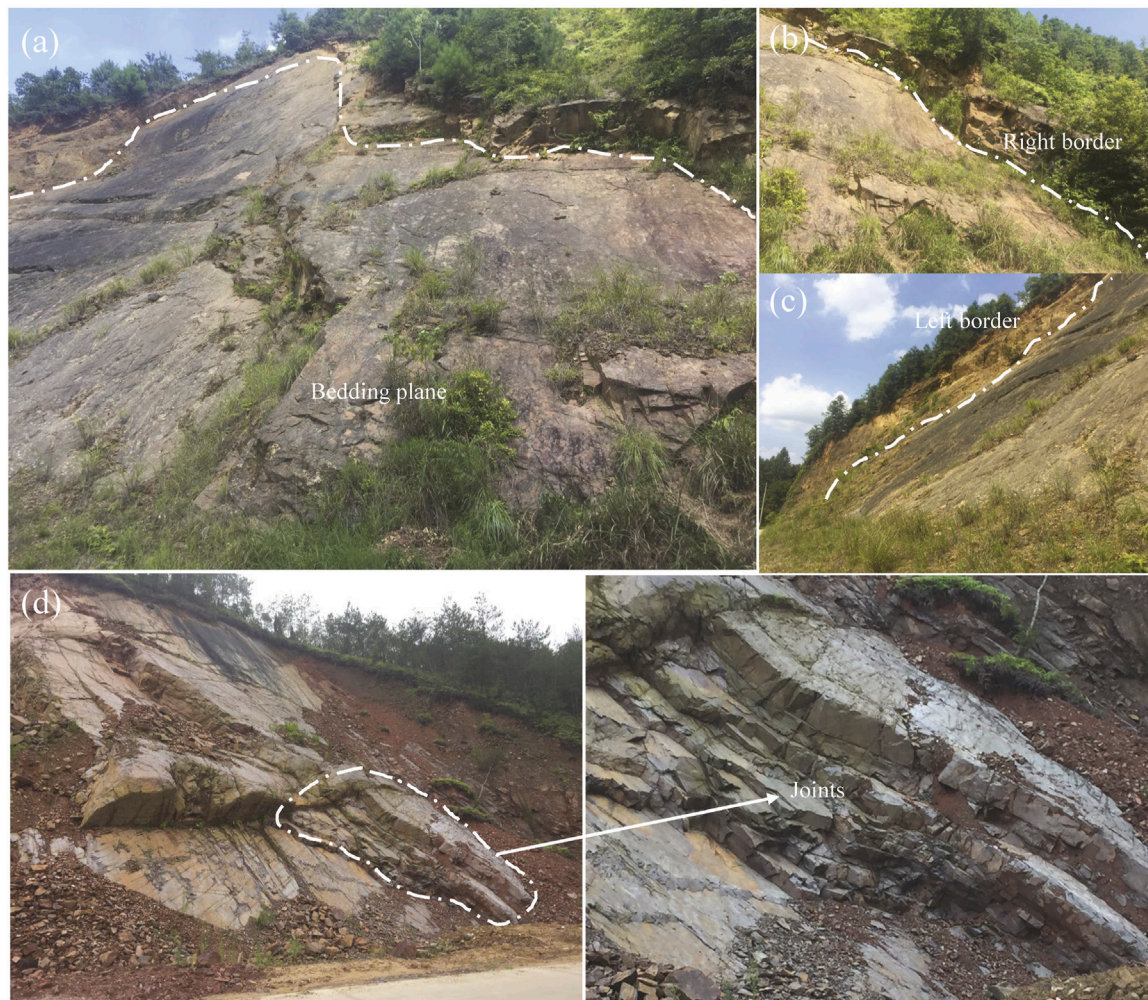
FIGURE 10 | Rockslides along a bedrock stratum in Ganzhou City: (A–C) Slope failure along a bedding plane in sandstone, X824 County Road. (D) Metamorphic slope near the Xinwuxiacun Village road.
