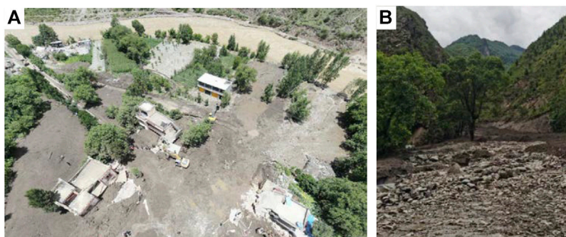
FIGURE 1 | Site photos of the Chenghuangmiao Gully debris flow disaster at the outlet ( https://720yun.com/t/38vksbpygp9?scene_id=50391102 ). (A) Buried houses and farms and (B) large-sized cobbles flushed out from the gully (a photo by the authors).
