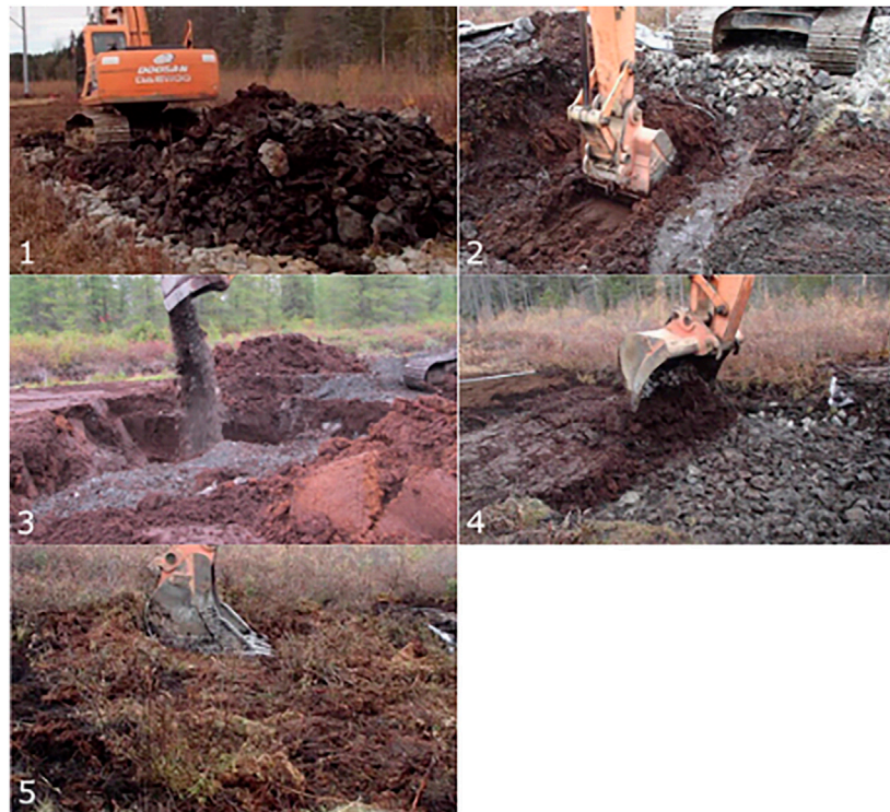
FIGURE 2 | Steps of the Burial Under Peat Technique: 1) excavation and stockpiling of the mineral material, 2) excavation of the underlying peat, 3) filling the pit with the mineral material, 4) covering the mineral material with excavated peat and leveling the soil surface with the adjacent peatland, and 5) revegetating of the peat surface with diaspores from adjacent peatland.
