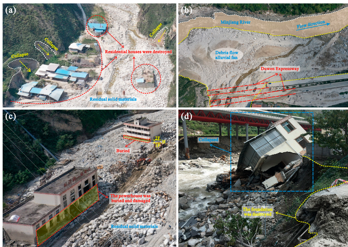
FIGURE 3 | Damage caused by debris flows in the “8-20” event: (A) buried houses in Banzi Gully; (B) the blocked Minjiang River and destroyed traffic facilities at the mouth of the Dengji Gully; (C) damage to the Banzi Gully Grade I Hydropower Station; and (D) destroyed buildings along the Minjiang River.
