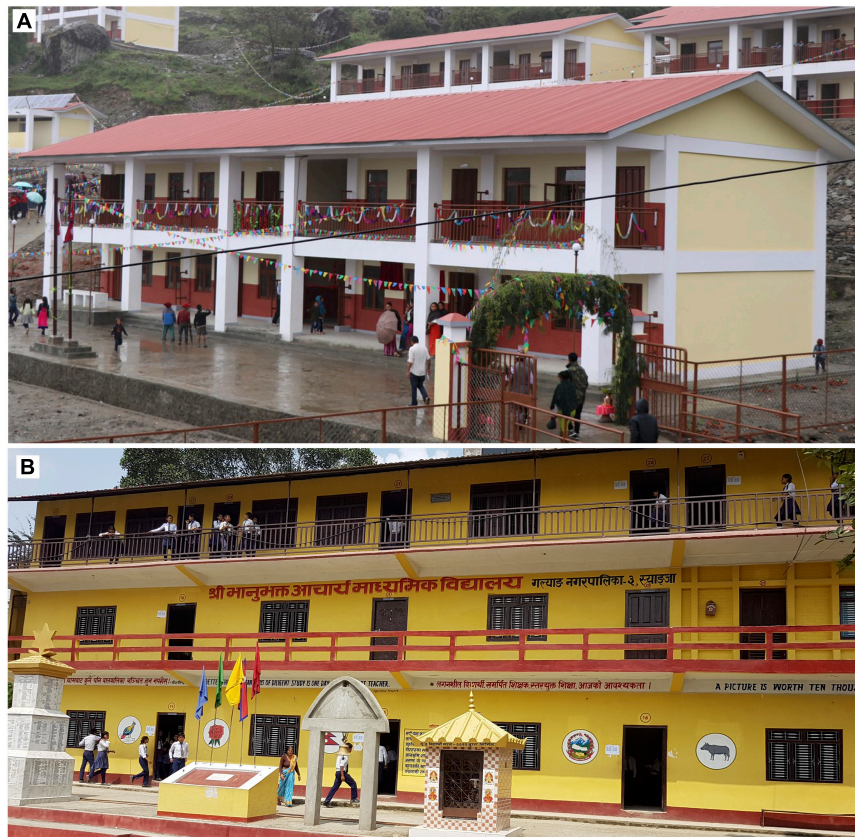
FIGURE 2 | School buildings participating in our program. (A) Shree Himalaya Secondary School in Barpak, Gorkha district. A reinforced cement concrete (RCC) building was newly constructed after the 2015 Gorkha earthquake. A total of 672 students study in the school. (B) Shree Bhanubhakta Acharya Secondary School in Galyang, Syangja district. RCC building, but the third story is not cemented: it is brick, with tin roof on top. A total of 925 students study in this school.
