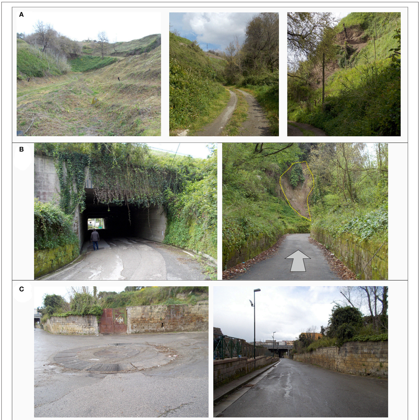
FIGURE 7 | Photographs of the different sectors of the studied watershed: (A) hilly sector with hollows and partly-natural channels, and soil slips along the slopes; (B) intermediate sector with a tunnel passing under the highway, and a drainage channel transformed in a road for connecting the urban center; the dashed line highlights the scar of a shallow landslide triggered by intense rainfalls; (C) lower and fully urbanized sector.
