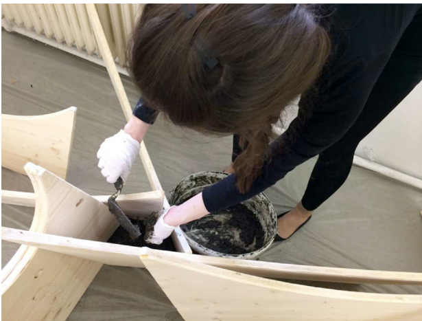
FIGURE 8 | Polymer concrete pouring.
