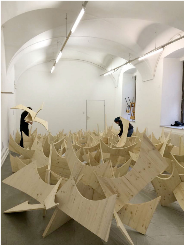
FIGURE 7 | The pre-assembled node modules act as lost formwork.
