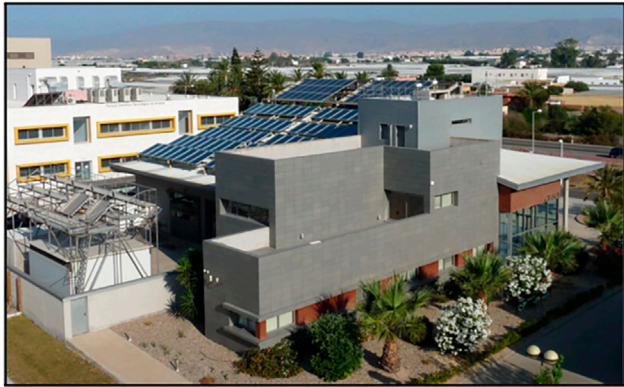
FIGURE 1 | Backside picture of the CIESOL building where the photovoltaic field and the field of solar collectors are visible in the rooftop.
