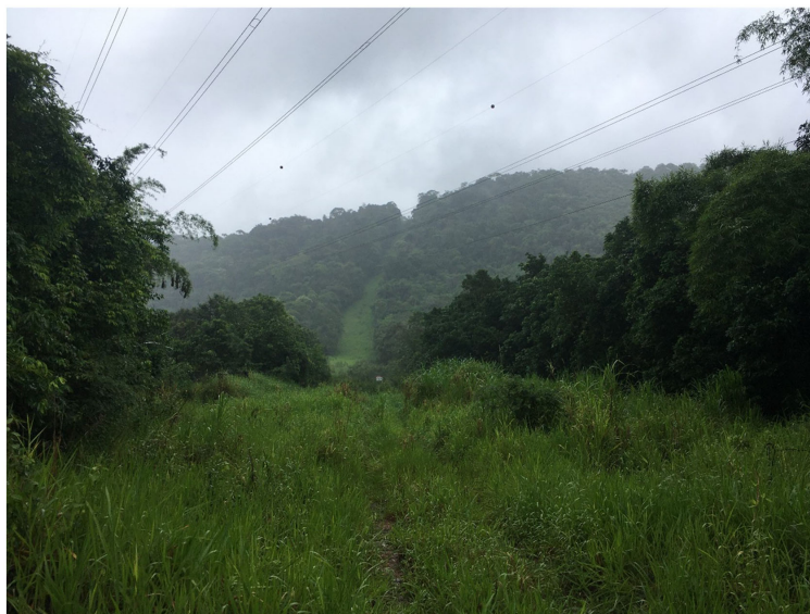
FIGURE 3 Photo of a right of way strip over the subterranean oil and gas pipeline traversing Haras de Flandria farm. The grassy vegetation over the strip was about 40 cm high at this time. High-tension electric power lines can be seen traversing over the strip.
