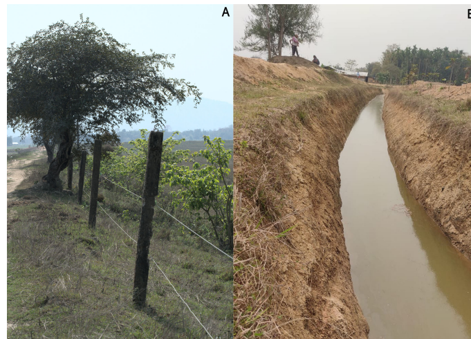
FIGURE 1 (A) Solar fence in Agorotoli range of Kaziranga National Park; (B) elephant-proof trench in Bokial range of Nabor Doiguring Wildlife Sanctuary.
