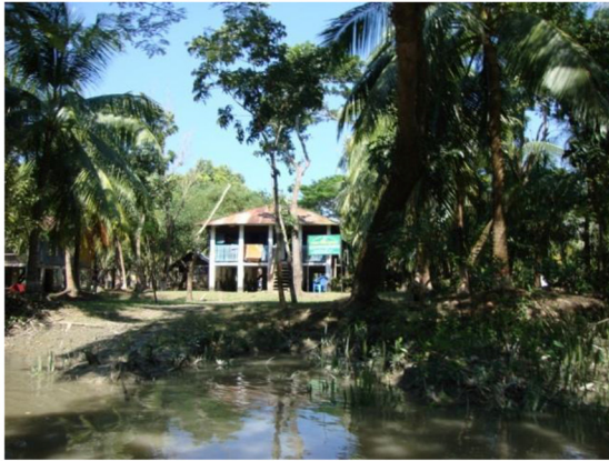
A Cyclone shelter in Muslimpara village on one of the islands.
