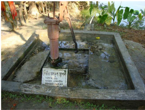
C A deep tube well installed by Coast Trust NGO for the villagers to get fresh drinking water (Muslimpara village).
