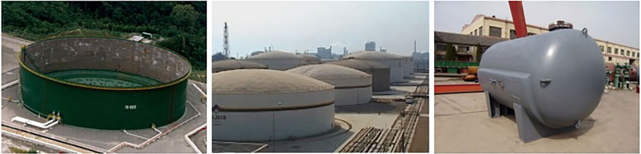
FIGURE 3 | Types of storage tanks from left to right (floating top vertical, horizontal, and fixed top vertical).
