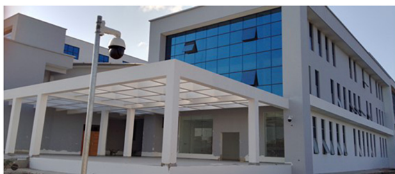
The just-completed EACoECVS Multipurpose Building
